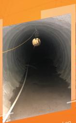
50 year-old steam tunnel on the University of Pittsburgh campus structurally rehabilitated with Geokrete<sup>®</sup> geopolymer
