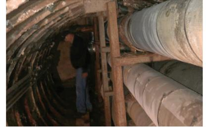
*Severe corrosion threatened the structural integrity of the old steam pipe.*
