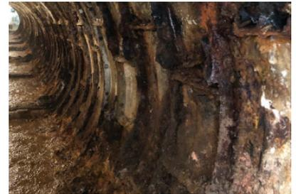
*The old piping and conduit was removed prior to relining the tunnel with QLS GeoKrete.*
