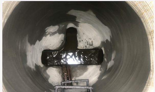
Manhole lined with QM-1s Restore and ready for Structure Guard epoxy coating for corrosion protection.
