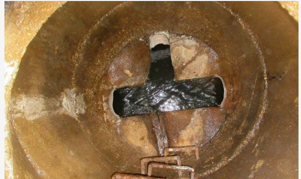
Typical manhole condition prior to lining with QM-1s Restore.
