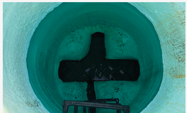
Structure Guard 100% solids epoxy was applied at 125 mils, to provide corrosion protection.
