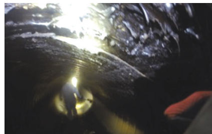
Pipe before cleaning, prep and lining.
