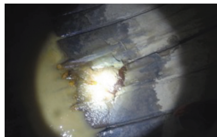
Example of corrosion and I/I before being lined with GeoKrete.
