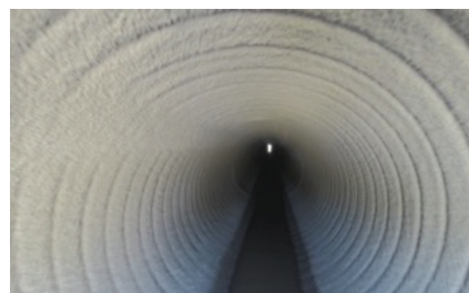
Pipe immediately after being lined with GeoKrete.
