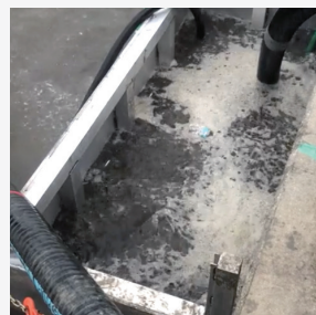
Daily dewatering was necessary due to outfall's proximity to the intracoastal waterway.
