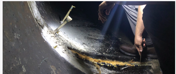
Leaks at the pipe joints were prepped and sealed with I&I Guard-PRF.
