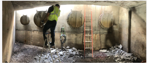
Clear evidence of concrete delamination in the D-4 Pump Station.
