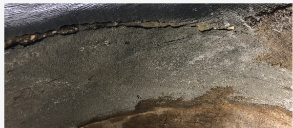
Cracks reveal failed cementitious liner from original project.
