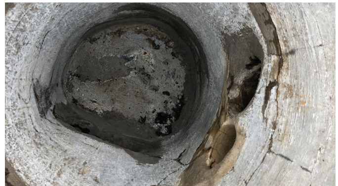
Before lining - cracks and voids are noticeably visible in this leaking manhole.
