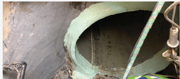
I&I Guard-PRF was applied to fill voids and cracks in manhole and pipe entry points.
