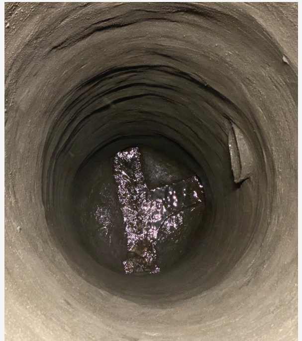
Prior to the application of Structure Guard, a 1" layer of AluminaLiner was applied for structure reinforcement.
