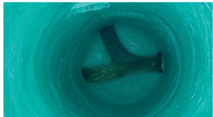
Rehabilitated manhole after being lined with underlayment of AluminaLiner and topcoated with Structure Guard.
