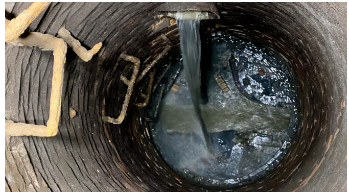
Deteriorating and exposed brick manhole with actively flowing service line.
