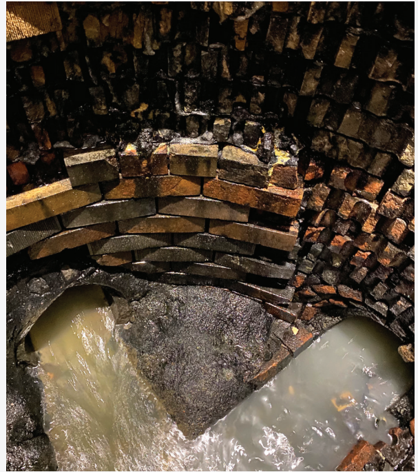
The old manhole had deteriorated to the point where many bricks were missing, corroded and falling apart. A collapse was imminent.
