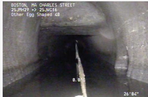
*“Boston Water and Sewer Commission completed a one year post inspection of the West Side Interceptor and the GeoKrete Geopolymer liner is still in the same condition as the day it was installed. The Commission is pleased with the work done by Quadex Lining Systems to structurally rehabilitate this interceptor sewer.” — Irene McSweeney, Boston Water and Sewer Commission*
