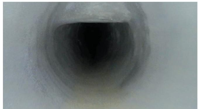
*After: 1.75" of QLS GeoKrete was spray-applied to the non-round areas of the tunnel and delivered the required structural and corrosion protection.*
