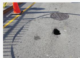
*Excessive I & I caused undermining of the street.*
