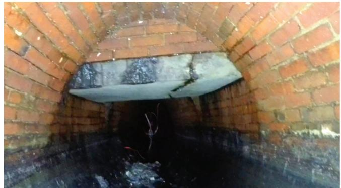
*Before: The effects of age and corrosion caused the brick sewer to leak in critical sections of this tunnel, including three headwall obstructions.*
