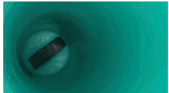
Completed manhole after Structure Guard® spray-applied and troweled to a smooth finish.
