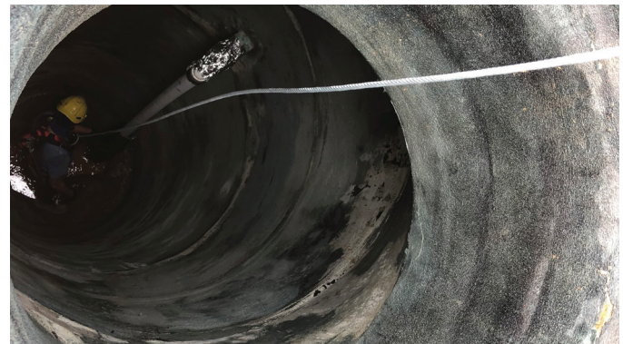
Manhole cleaned and prepped, awaiting structural and corrosion protection.
