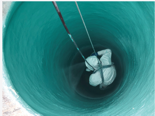
Structure Guard can be applied up to 250 mils per pass.
