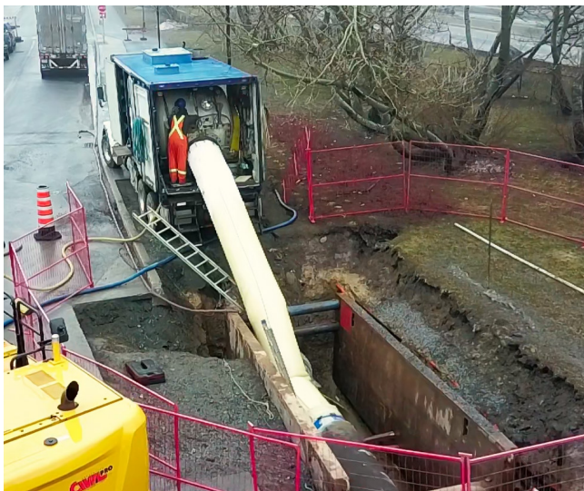
Project completion through CIPP required only minimal excavation, reducing costs and ensuring a faster return to service.
