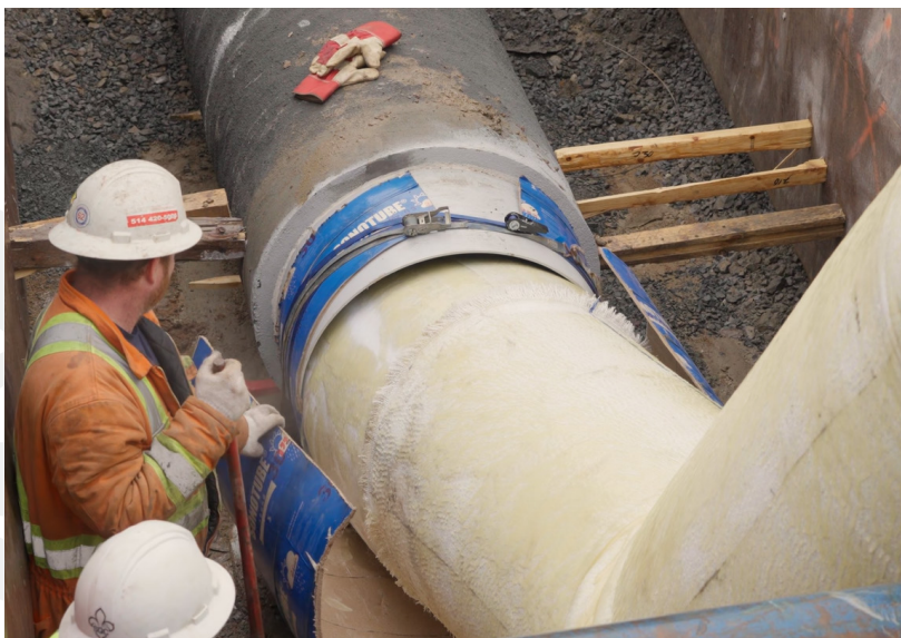
The liner installation portion of the work was completed in only five days.
