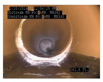
Depending on the level of pipe contamination, the crew utilized cleaning tools from traditional Level 1/Level 2 nozzles to heavy-duty Warthog Magnum Switcher and descaler nozzles. Alongside these cleaning efforts, the team gathered condition assessment data which would be used to determine the required amount and kind of rehabilitation necessary for each section of piping. Once these cleanings
