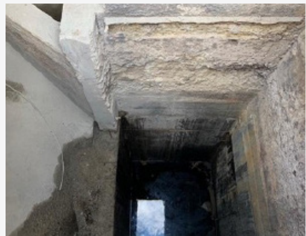
Years of exposure left the interceptor pipeline and siphons in a highly deteriorated condition.
