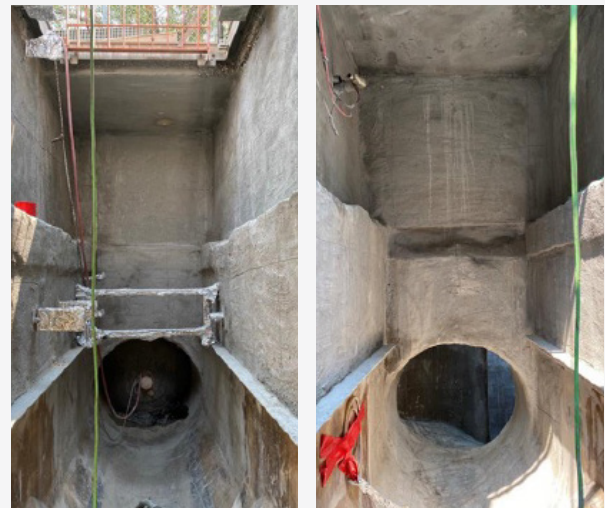
Years of exposure left the interceptor pipeline and siphons in a highly deteriorated condition.
