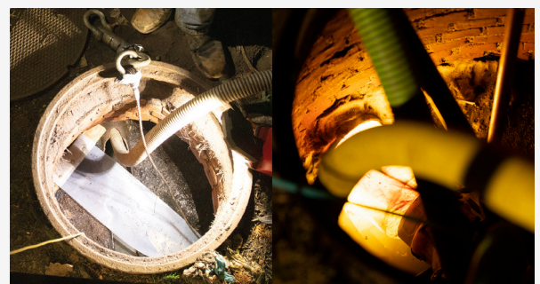
A glider foil, installed prior to inserting the UV liner, reduces friction during liner pull-in process.
