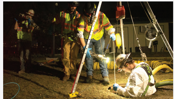
Vortex Services installation crew inserting the UV light chain into the manhole to begin the UV curing process.
