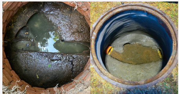
Manholes were deteriorated and leaking.
