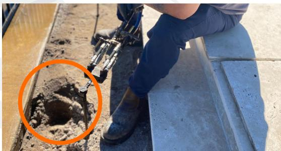
*As technician injects I&I Guard - SSF into void behind seawall, signs of soil erosion were evident.*
