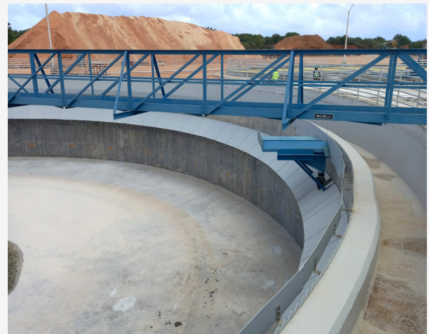
Newly constructed clarifiers were coated with SEL-80 as preventative maintenance measure
