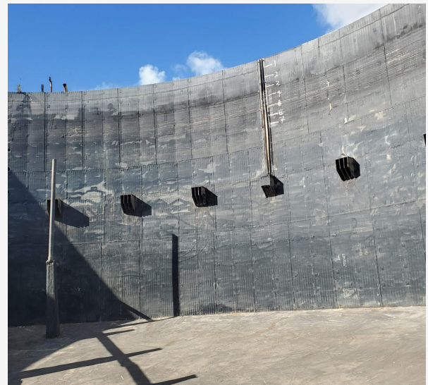
Several Tanks with failed T-Lock were stripped and then coated with Parsonpoxy SEL-80 100% solids epoxy
