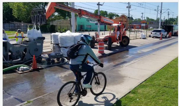
Vortex was able to rehabilitate the 60" sanitary sewer line running beneath a section of the City's light rail train tracks.
