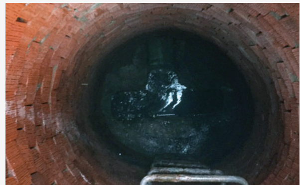
Manhole condition prior to GeoKrete geopolymer application.
