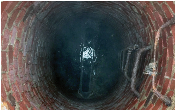
Manhole condition prior to application of GeoKrete Geopolymer.
