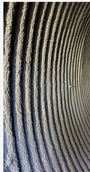
The wall of the culvert before having GeoKrete geopolymer spray applied.
