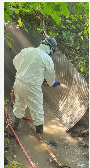
The wall of the culvert before having GeoKrete geopolymer spray applied.
