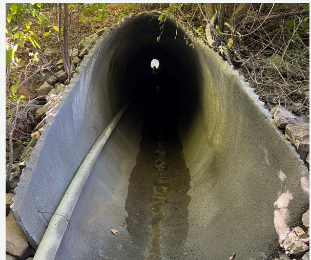
The culvert pipe was fully rehabilitated due to the innovative and efficient spray-on application of GeoKrete geopolymer.
