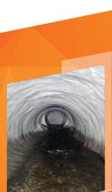
GeoKrete<sup>®</sup> geopolymer secured to rehabilitate a 60 year-old CMP storm culvert beneath major Connecticut highway
