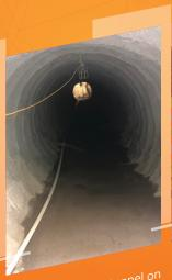
50 year-old steam tunnel on the University of Pittsburgh campus structurally rehabilitated with Geokretes geopolymer
