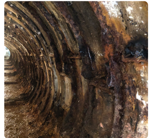
The old piping and conduit was removed prior to relining the tunnel with QLS/GeoKrete.
