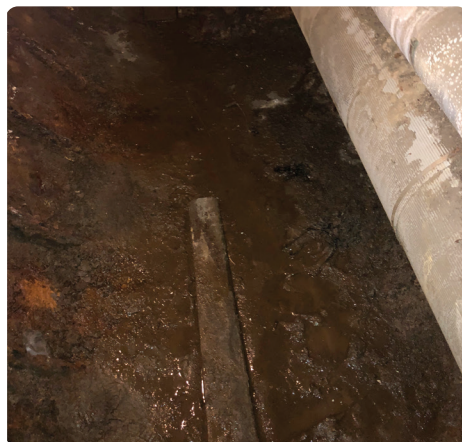
The original rounded floor of the steam tunnel was not only slippery, it was difficult for maintenance crews to gain purchase.
