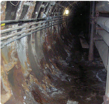
Condition of the tunnel and placement of the conduit prior to removal and rehabilitation.
