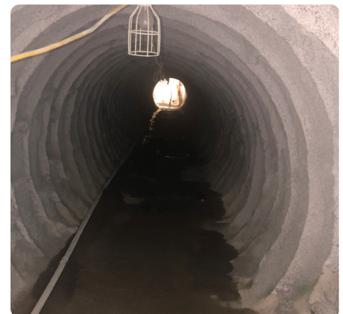
After 1.5" of QLS GeoKrete was spray-applied to structurally renew the deteriorating steam tunnel.
