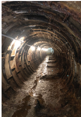
Condition of steam tunnel proper to QLS/GeoKrete® installation.
