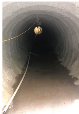
After the steam tunnel is lined with GeoKrete and floor leveled with Quad-Flow.
