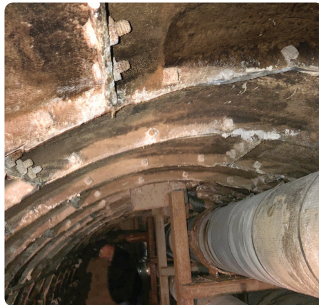
Severe corrosion threatened the structural integrity of the old steam pipe.
