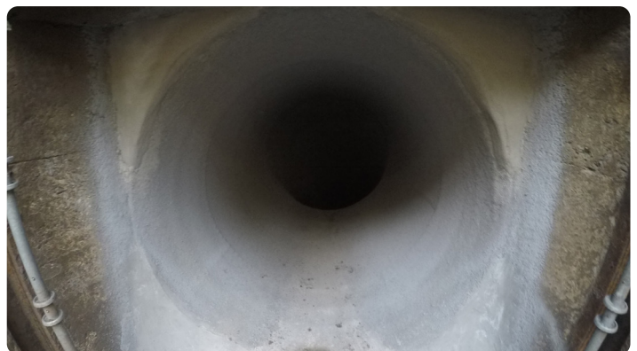
GeoKrete Liner - Structural renewal and restored flow capacity.
