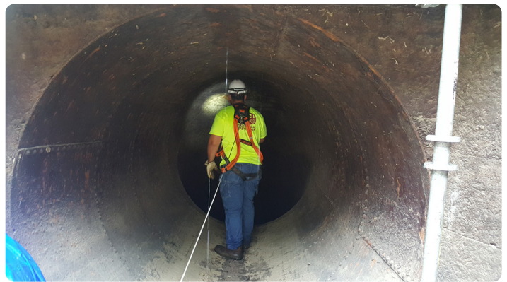
Peering down the steep slope of penstock.
