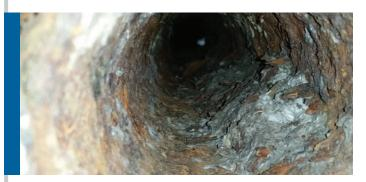
**BEFORE:** In many cases, water and sewer pipes that appear to be beyond repair can be CIPP lined and fully rehabilitated.
