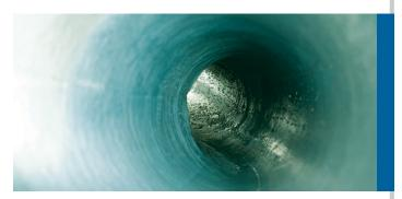
**AFTER:** CIPP lining systems combine liner materials with resins designed and formulated to address the demands of your piping system.
