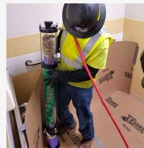
*Inserting CIPP liner into branch line located inside apartment.*
