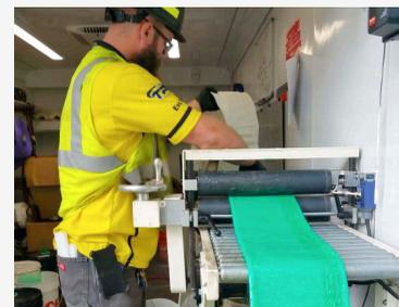
*Wet-out of CIPP liner to rehab stack and branch lines.*
