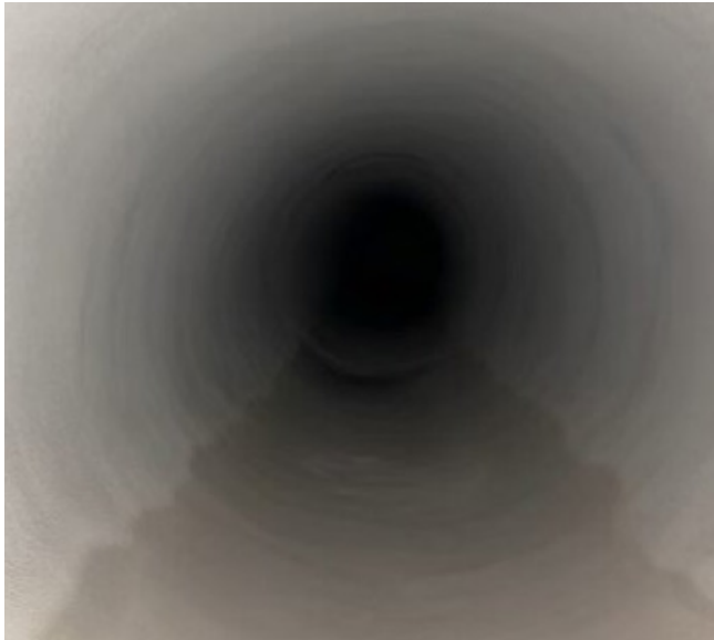
The rehabilitation eliminated the corrugations and created a new, structurally-sound tank.
