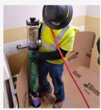
Inserting CIPP liner into branch line located inside apartment
