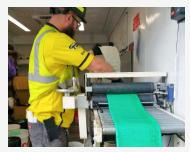
Wet-out of CIPP liner to rehab stack and branch lines.
