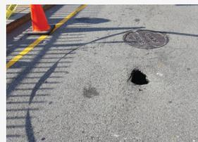
*Excessive I & I caused undermining of the street.*
