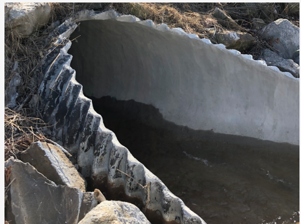
GeoKrete can be hand or spray applied depending on shape and condition of the pipe or structure.
