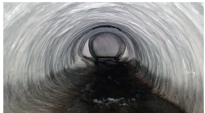
Culvert after full structural rehabilitation using GeoKrete geopolymer.
